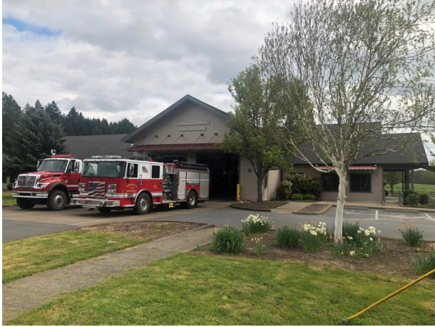
Locke Fire Station with Tender 146 and Fire Engine 136
